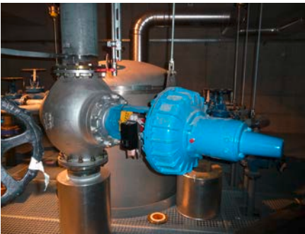
6N-Armatur für ND-Dampf-System 6N valve for low-pressure steam system
